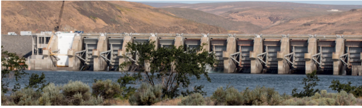
Work on Wanapum Dam's 12 gates took 3 years and included full class A containment, lead removal, and coating with a moisture-cured coating system.
