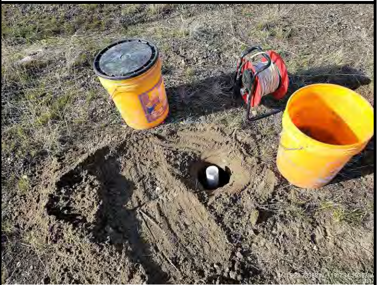
View of infiltration test at Boring B-14 / IT-4
