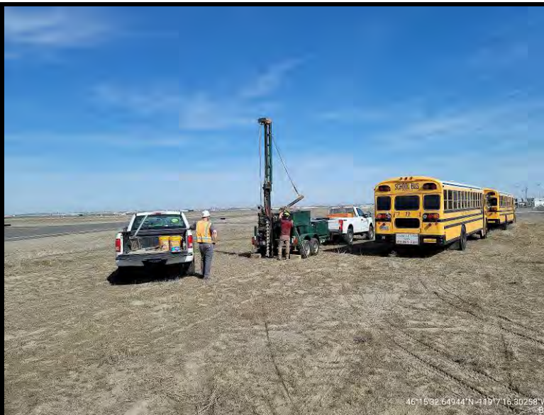
View of Boring B-9 looking north
