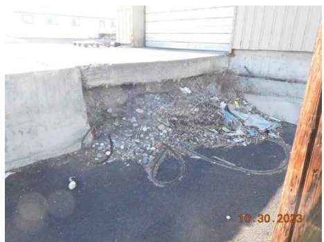
WH7B4 SOUTH RAMP AT NORTH SIDE
