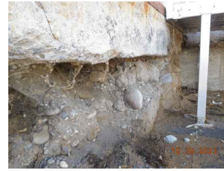
WH8B4 EXIST. SLAB EDGE NORTHSIDE.
