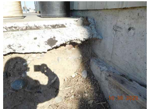
WH4B1 RAMP SLAB AT WH WALL.
