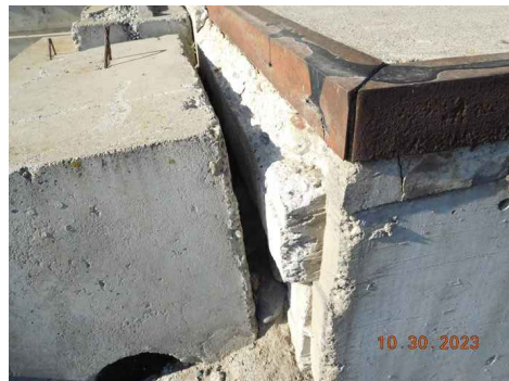
WH1B4 EXIST. CONDITION
