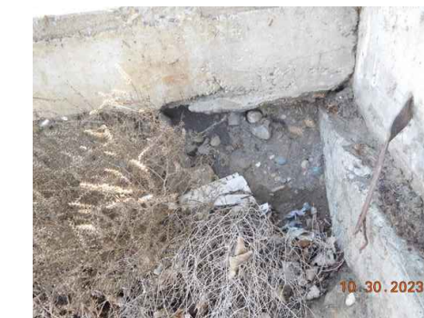
WH7B4 RAMP SLAB AT WH WALL.
