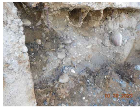
WH8B4 EXIST. CONDITION NORTHSIDE UNDER DOCK SLAB.
