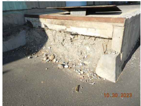
WH8B4 EXIST. CONDITIONS SOUTHSIDE OF DOCK.
