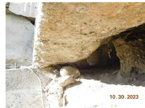
WH3B4 UNDERSIDE EDGE OF RAMP AT WH WALL.
