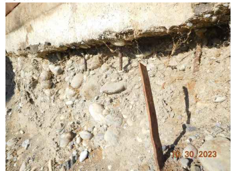
WH8B4 EXIST. SLAB EDGE AT SOUTHSIDE.
