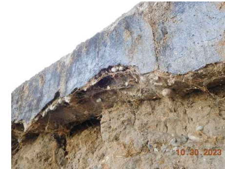
WH8B4 UNDERSIDE EDGE OF RAMP.
