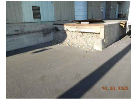
WH8B4 EXIST. CONDITION SOUTHSIDE.
