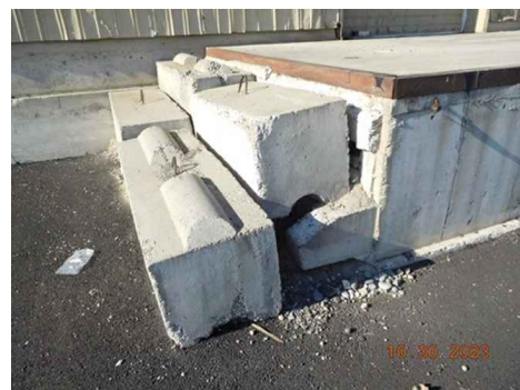
WH1B4 EXIST. CONDITION.
