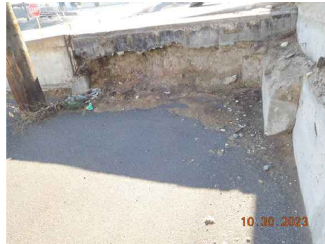
WH8B4 NORTHSIDE OF SOUTH RAMP EXIST. CONDITIONS.
