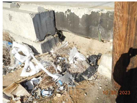
WH2B4 EXIST. CONDITION
