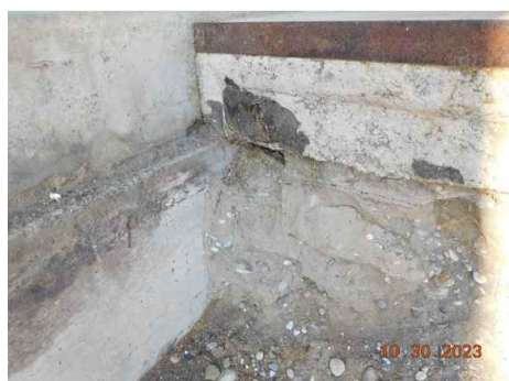
WH8B4 DOCK SLAB AT WH WALL SOUTHSIDE.
