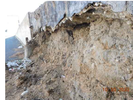
WH8B4 UNDERSIDE EDGE OF RAMP.
