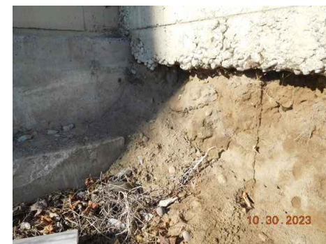
WH6B4 LOOKING UNDER SLAB EDGE AT WALL
