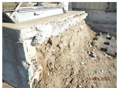
WH4B1 END OF DOCK EXIST. CONDITIONS.
