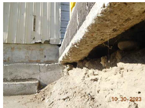
WH3B4 UNDERSIDE OF EDGE OF RAMP
