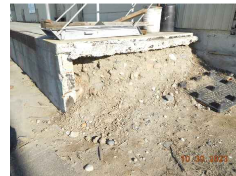
WH4B1 END OF DOCK EXIST. CONDITIONS.
