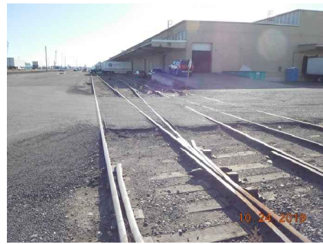
TRACK 411 & 416 LOOKING EAST AT WH3
