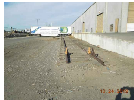
TRACK 451 LOOKING WEST AT T1-79
