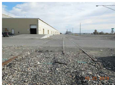
TRACK 451 & 452 LOOKING EAST AT WH7
