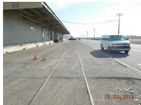
TRACK 418 LOOKING EAST AT WH5
