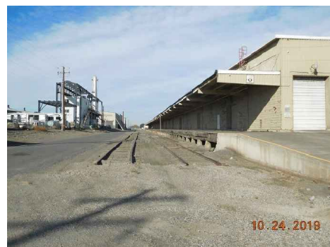
TRACK 451 & 452 LOOKING WEST AT WH8
