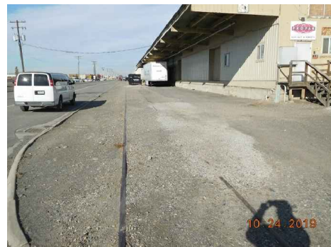
TRACK 418 LOOKING WEST AT WH5
