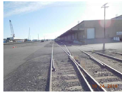
TRACK 411 & 416 LOOKING EAST AT WH4
