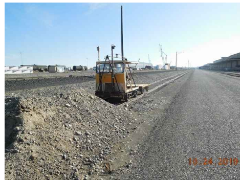
SPUR TRACK LOOKING EAST
