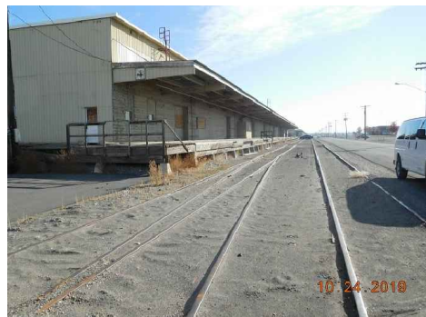
TRACK 418 & 420 LOOKING EAST AT WH4
