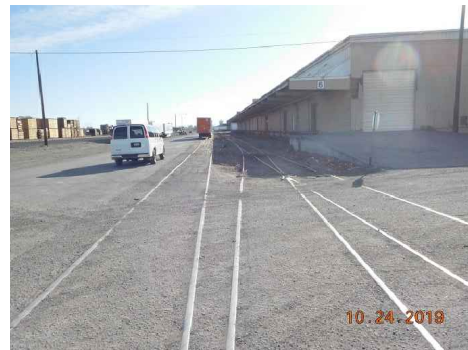
TRACK 411 & 416 LOOKING EAST AT WH6
