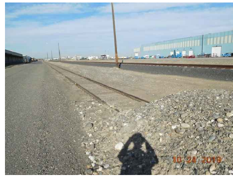
SPUR TRACK LOOKING WEST
