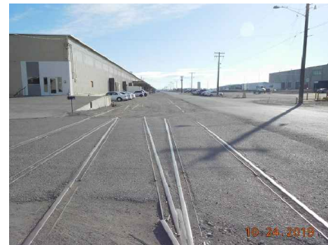
TRACK 418 & 420 LOOKING EAST AT WH3
