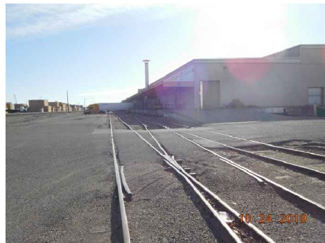
TRACK 411 & 416 LOOKING EAST AT WH5
