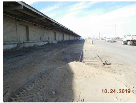
TRACK 411 & 416 LOOKING WEST AT WH3
