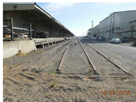
TRACK 451 & 452 LOOKING EAST AT WH8
