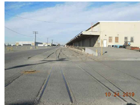
TRACK 418 & 420 LOOKING WEST AT WH3
