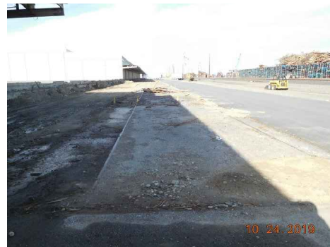
TRACK 411 & 416 LOOKING WEST AT WH6
