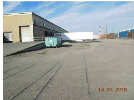
TRACK 411 & 416 LOOKING WEST AT WH5
