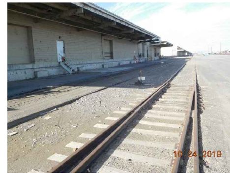
TRACK 411 & 416 LOOKING WEST AT WH4
