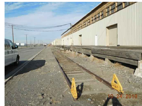
TRACK 418 LOOKING WEST AT WH6
