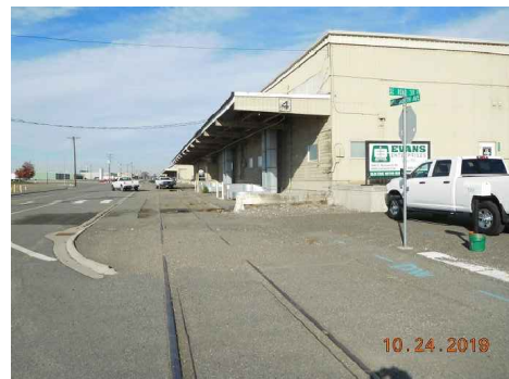
TRACK 418 & 420 LOOKING WEST AT WH4
