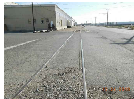
TRACK 418 LOOKING EAST AT WH6
