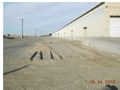
TRACK 451 & 452 LOOKING WEST AT WH7
