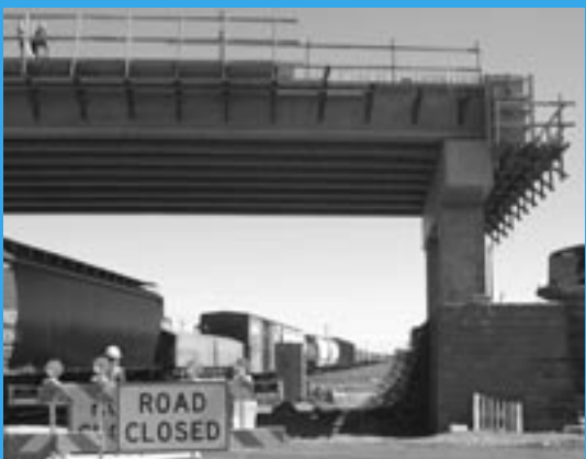
Train traffic is already able to run under the new overpass.
