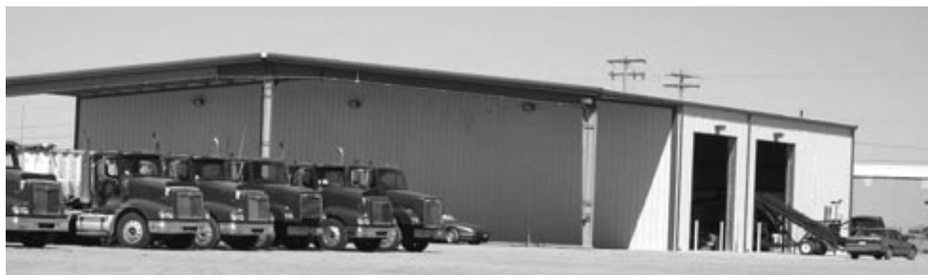
Easterday Farms' new building located on a Port of Pasco site includes a shop and space for its fleet of 20 trucks.
