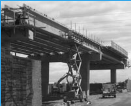
The new bridge structure of the Ainsworth Overpass is nearing completion.
