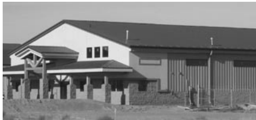
The Tri-Cities Airport Business Center is the new home of two local businesses and the first buildings in the new development. Gauntt Farms relocated its office/hangar from Kennewick.
